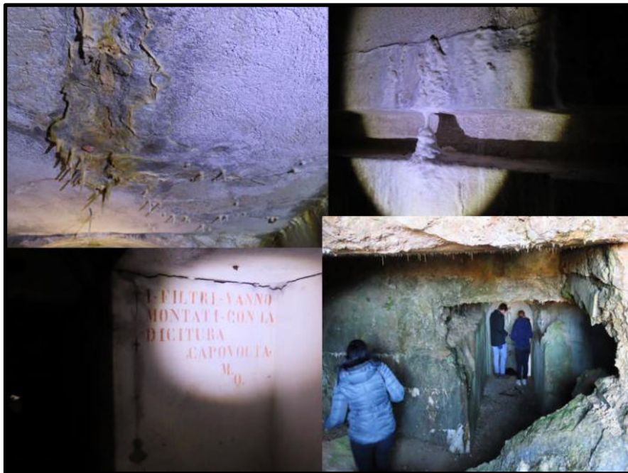
Figure 23.6: Inside the tunnels in Milanja (above Ilirska Bistrica)
