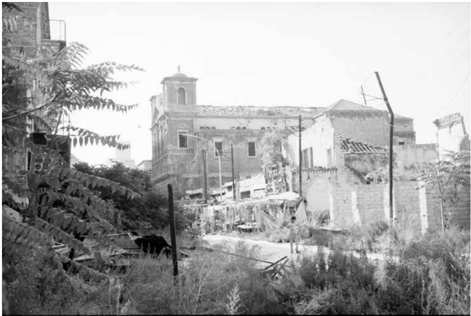
Fig. 10. Saint Joseph Church, Jesuit quarter (Achrafieh area) – at the time of the civil war (Photo © Archive of the Oriental Library, St. Joseph University.-Civil War Photo Collection).
