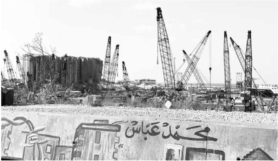
Fig. 1. The port of Beirut after the deflagration on 4 August 2020,(© Photo Daniela Dumbravă).
